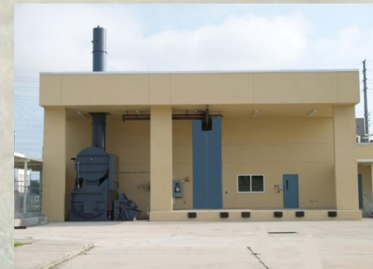
Necropsy & Incineration facility
