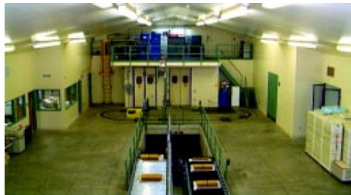
Facility process area
